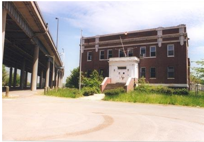
WAR Transmitter building, Jones Point, Alexandria VA
