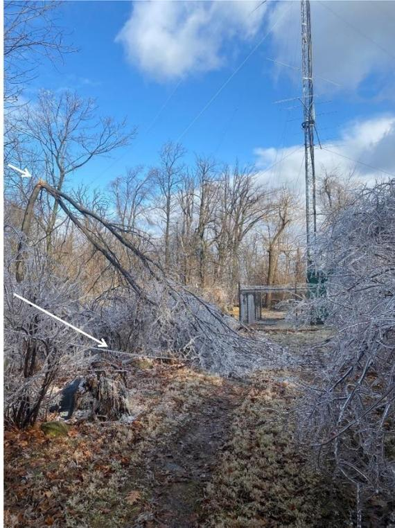
WARC inverted vee center mount detached, wires laying on 20/15/10 trapped dipole
